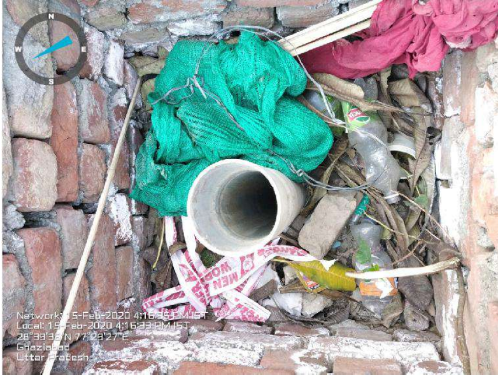
Sec-2 Existing Tubewell 2 in G- 3 Open
