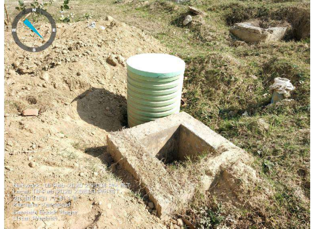
Sec-5 RWH Pit No 4 in WEF
