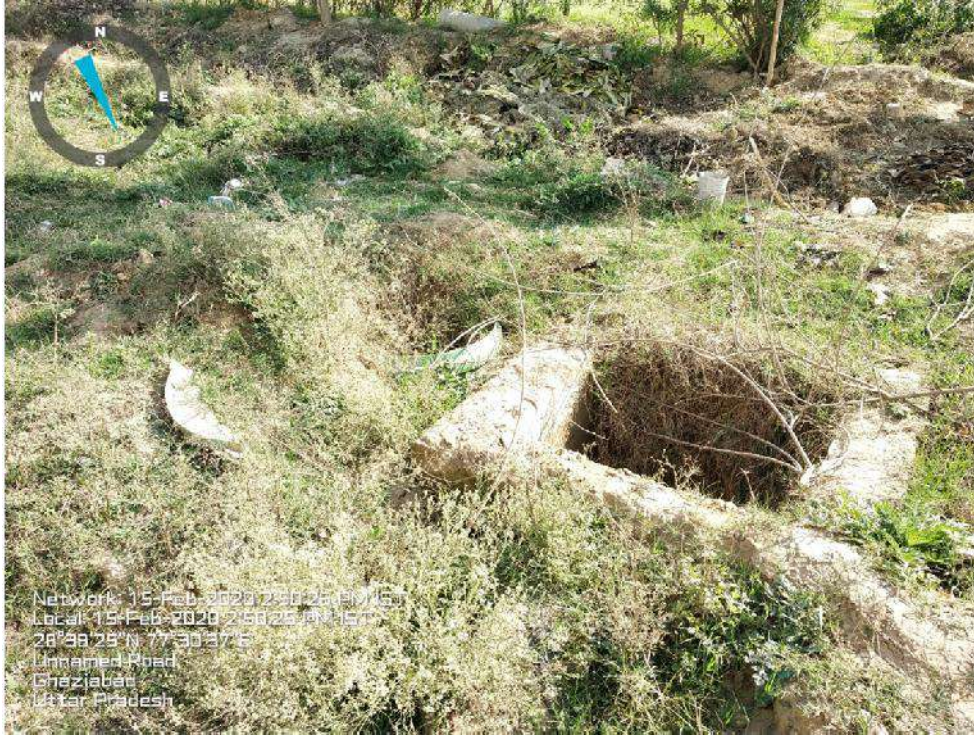
Sec-5 RWH Pit No 13 in WEF
