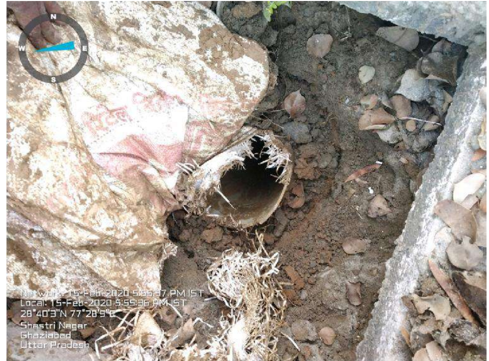
Sec-3 RWH Pit No 1 Boring in Gallaria
