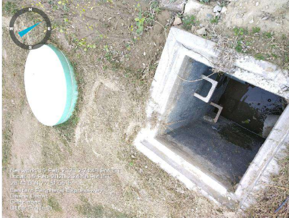
Sec-5 RWH Pit No 7 in WEF
