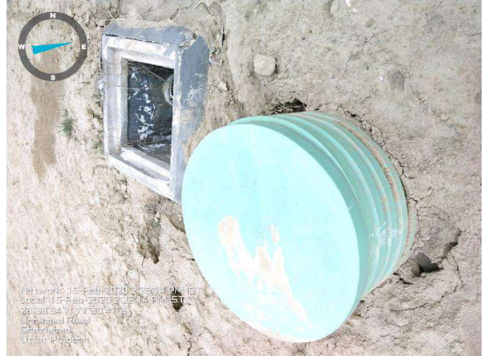
Sec-5 RWH Pit No 6 in WEF
