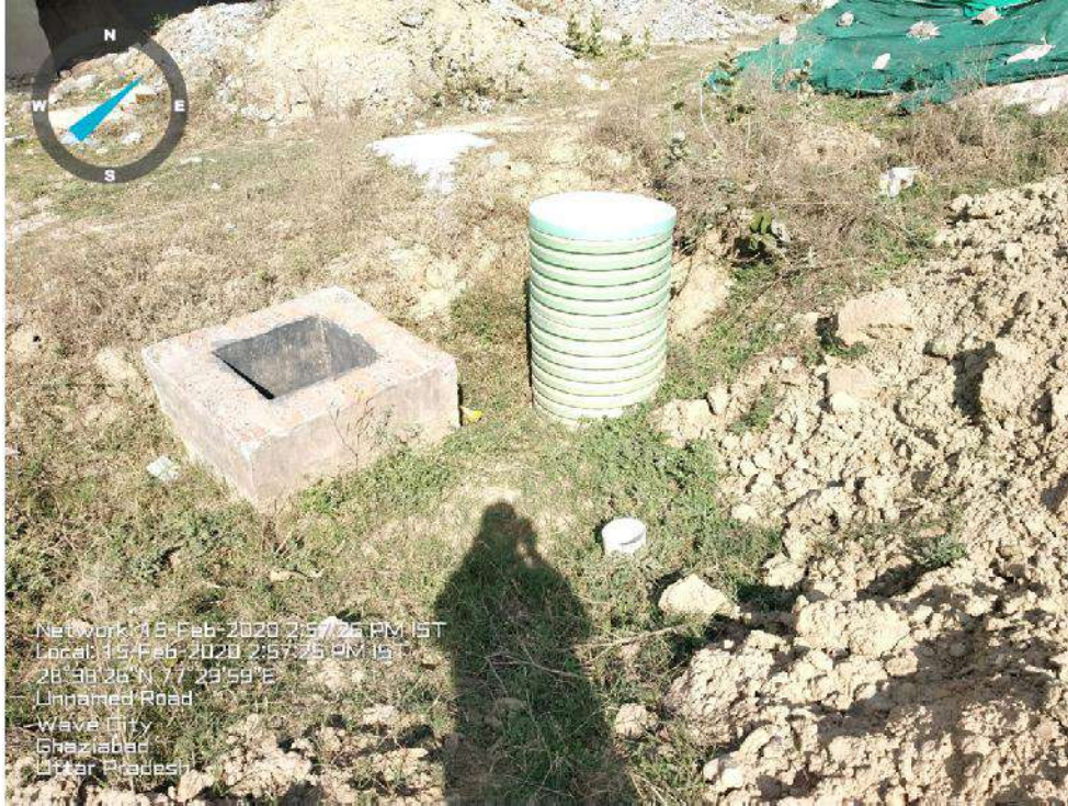
Sec-5 RWH Pit No 5 in WEF
