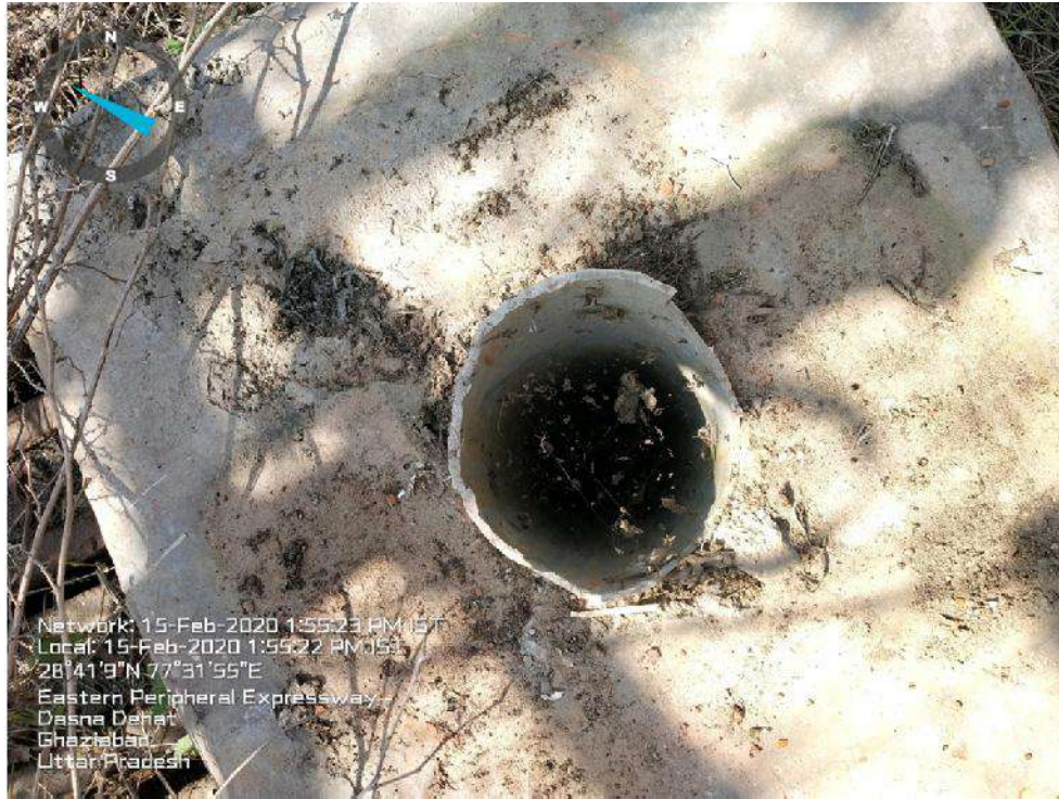
Sec- 5 Existing Tubewell in EWS Open
