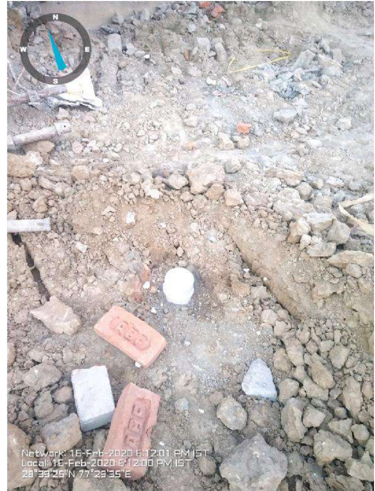
Sec- 2 Existing Tubewell 1475 Sealed
