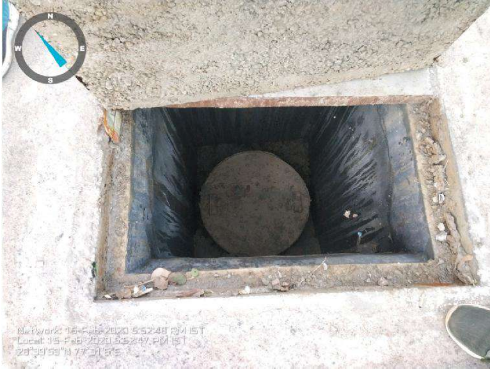
Sec-3 Filter RWH Pit No 1 in Gallaria
