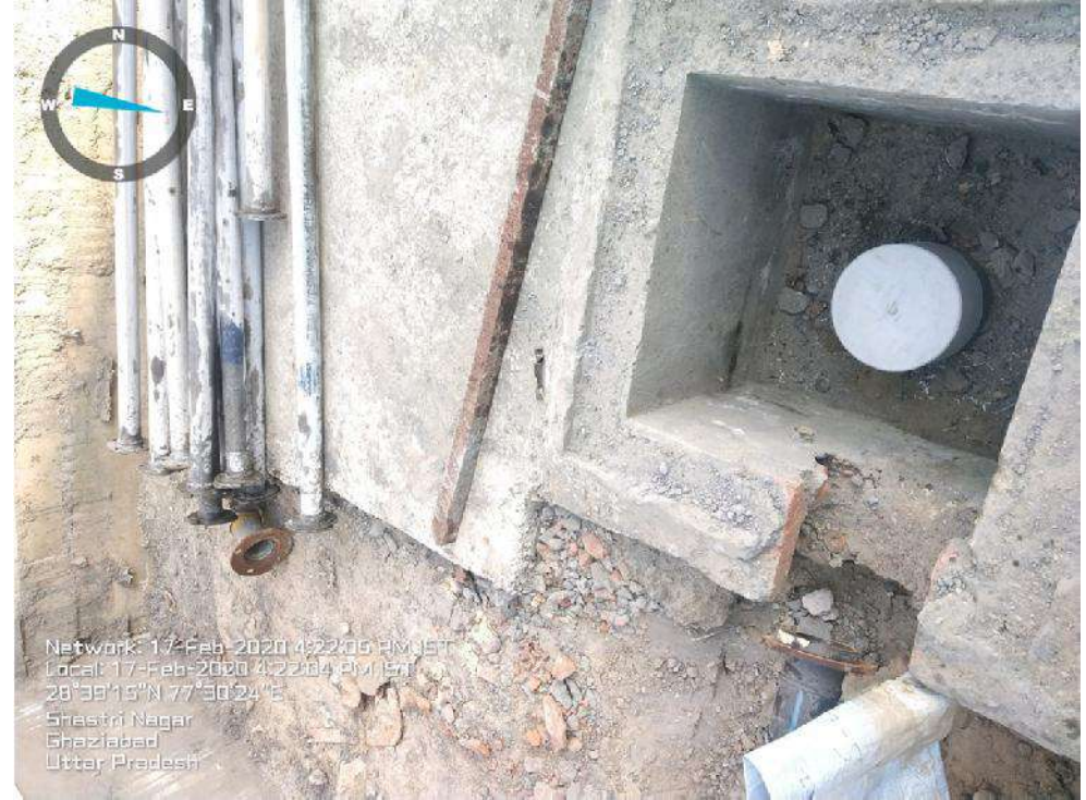
Sec-3 Existing Tubewell 2 in Galleria Sealed
