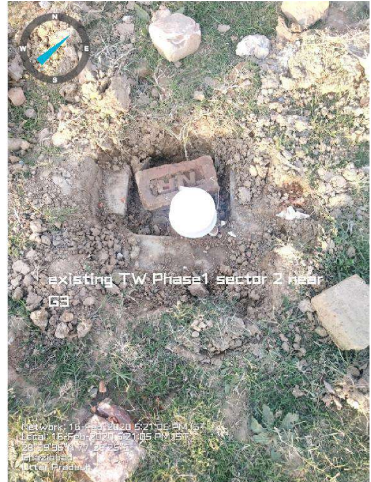
Sec-2 Existing tubewell 019N Sealed
