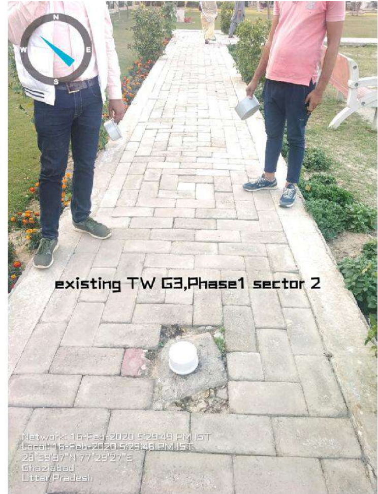
Sec-2 Existing Tubewell in G-3 Sealed
