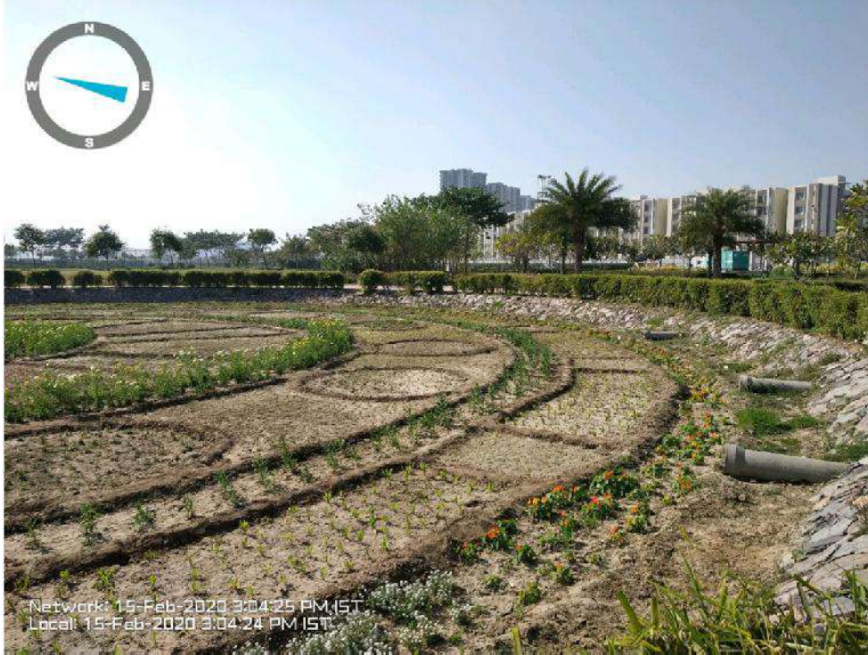
Sec-5 Recharge Pond 3
