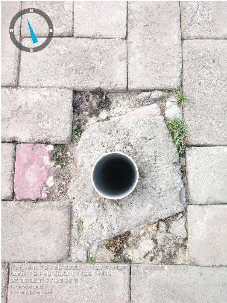
Sec-2 Existing Tubewell in G- 3 Open
