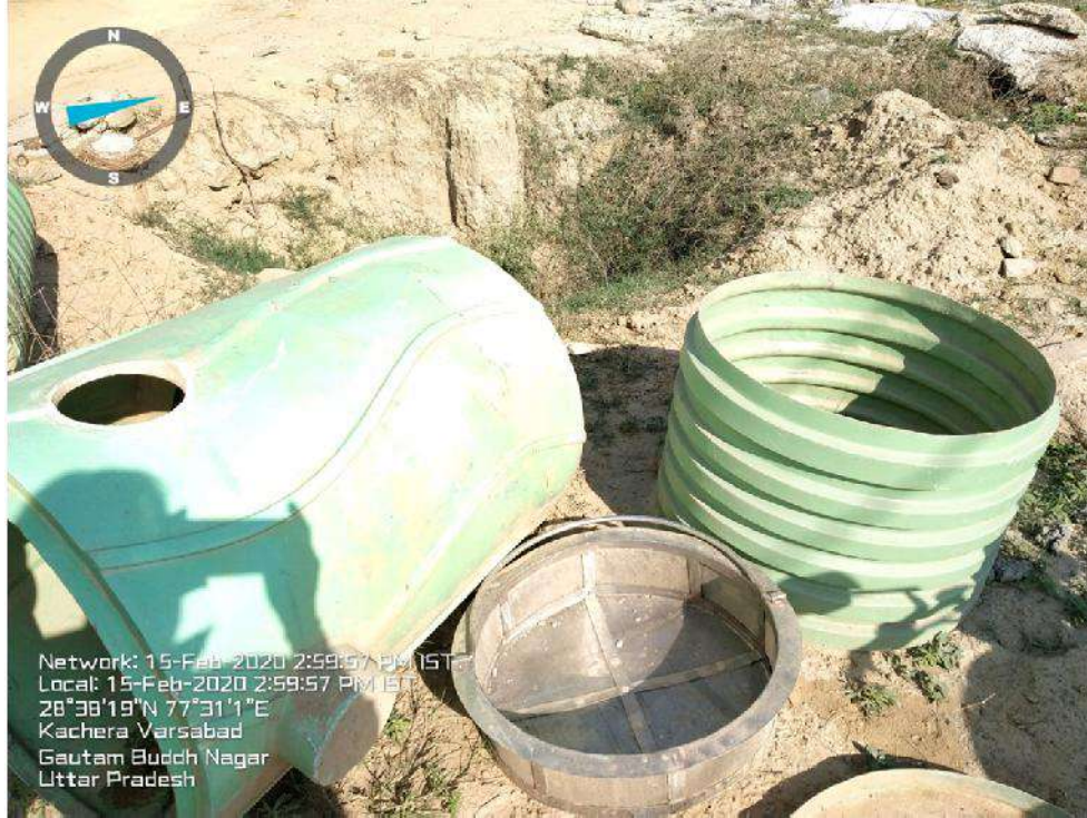
Sec-5 RWH Pit No 3 in WEF
