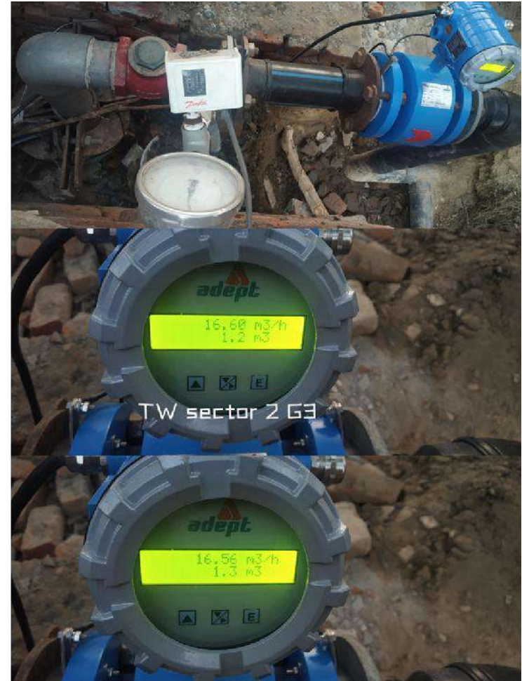
Sec-2 Tubewell in G-3 with Flow Meter
