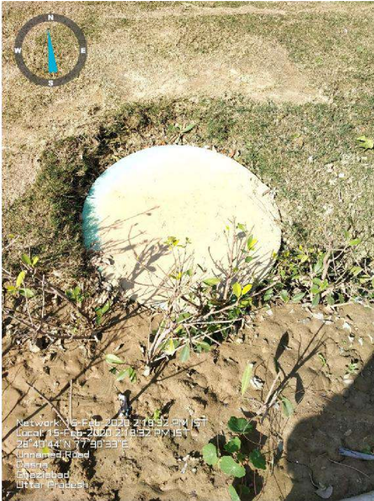
Sec-5 RWH Pit No 9 in WEF
