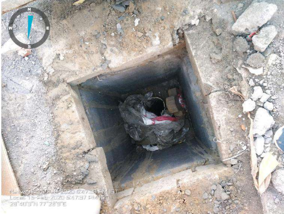
Sec-3 RWH pit No 3 boring in Gallaria
