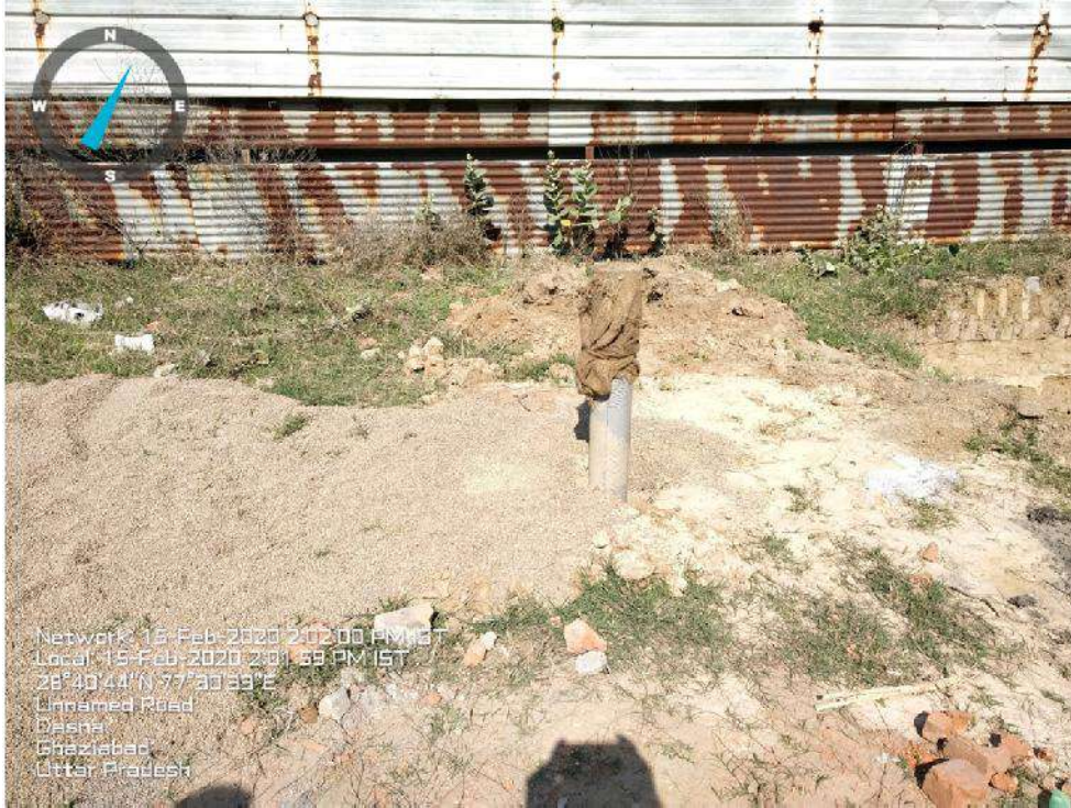
Sec-5 RWH boring in EWS
